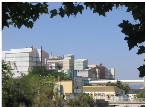
Figure 1. Axens Salindres Manufacturing Site
